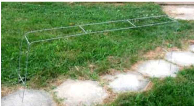
Mason Ladder Cut and Bent to Proper Shape
