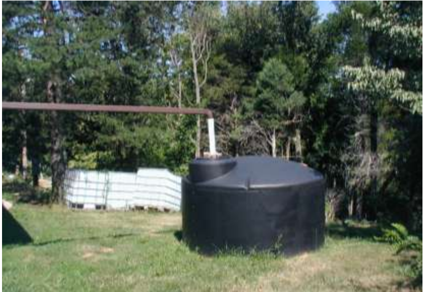
Now, That is Some Rain Barrel Paul! A 1300 Gallon Tank Being Filled by Garage Roof Runoff. (Also, You Must Have One Big Garage.)
